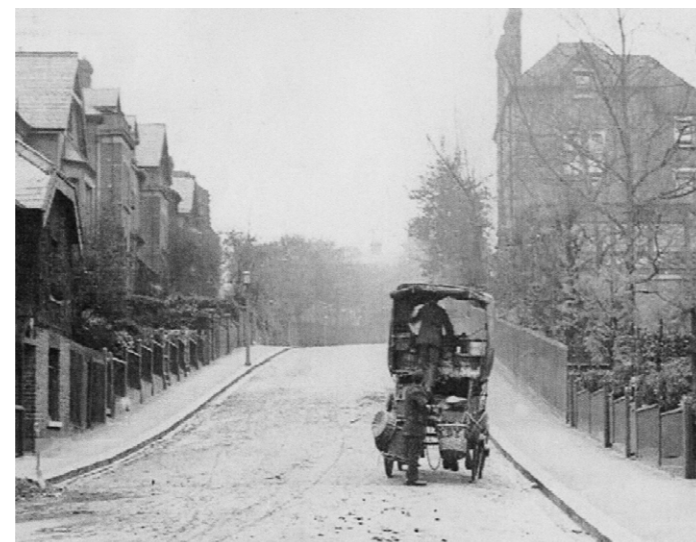
The top drawing shows Lewisham Hill by TM Baynes in 1823, with Mortimer's house on the right. These houses were occupied by minor professional people and Charles Mortimer was a clerk in the Postmaster General's personal office. The lower photo is of Blackheath Rise in Lewisham, taken around 1905
