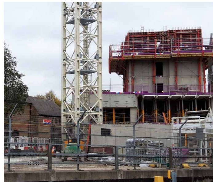
The Tesco tower starts to rise next to Lewisham station
