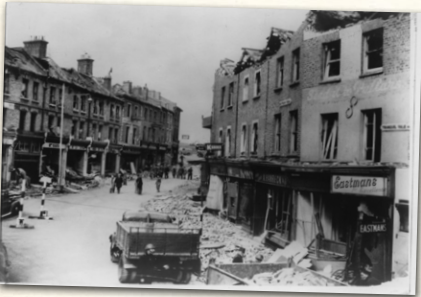
War damage in March 1945 when a V2 rocket hit Blackheath Grove
